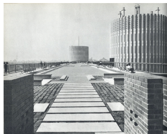
Figure 10: Palace Side Building (Nikken Sekkei, 1966)
